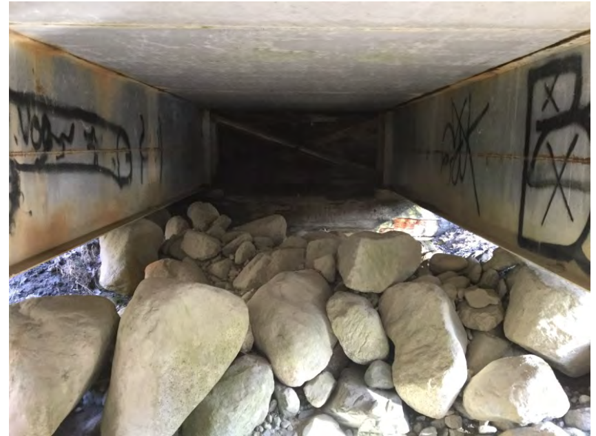
Left Bank Abutment when facing downstream
