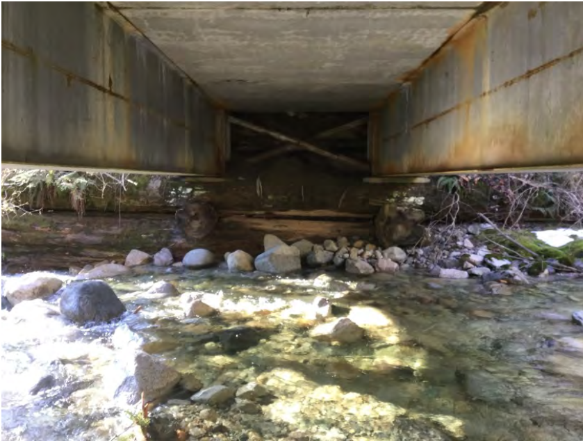
Right Bank Abutment when facing downstream
