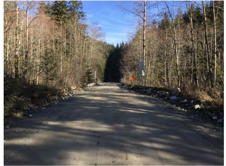
Approach from Right Bank when facing downstream
